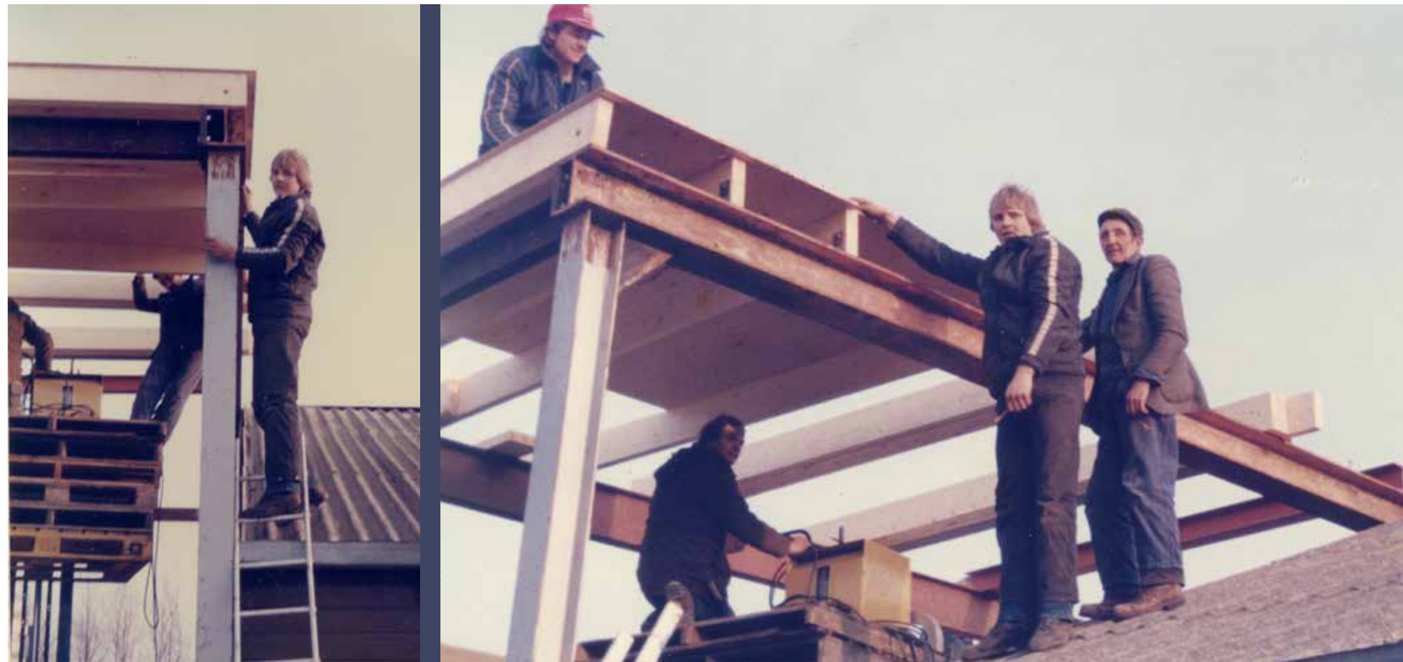
February 1985, the building of a raised barn to facilitate the new fibre press.
